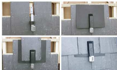
Step 4: Cut slates around the hood of the SolarFlash as per Page 4.
